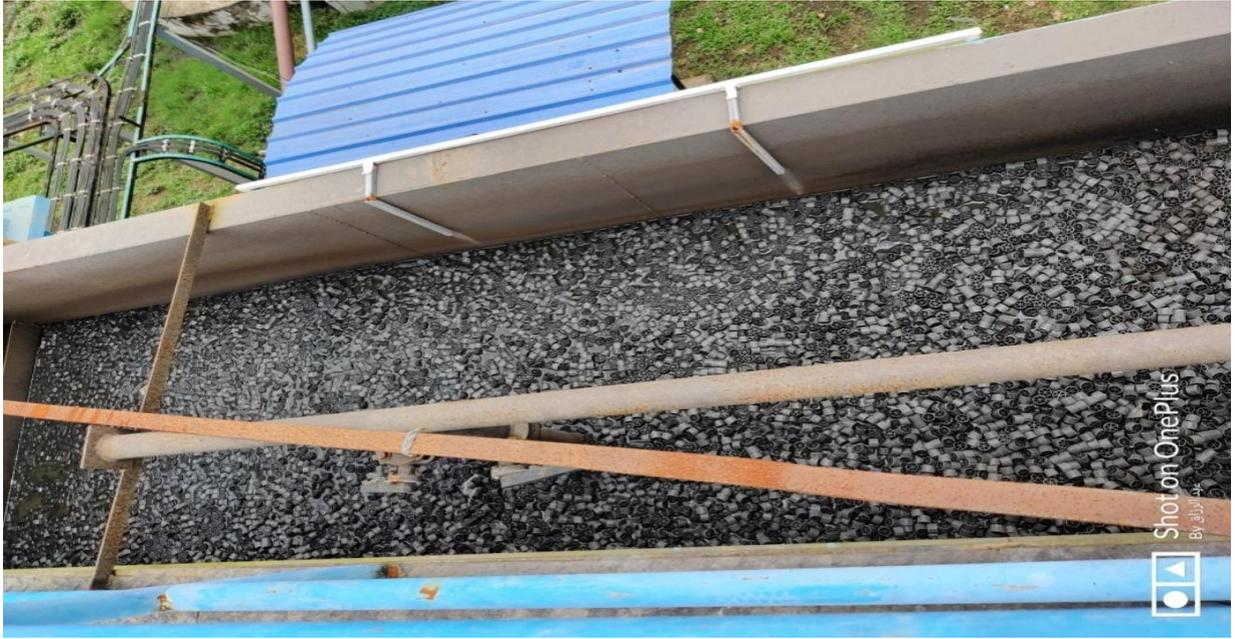
Fig. 18.17 Moving Bed Bio Reactor in the Septage treatment plant, Willingdon island
