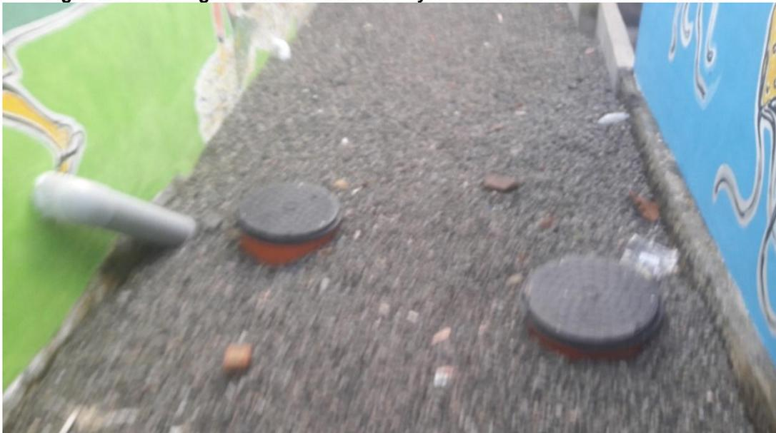
**Fig.18.21 Manholes in the pipe lines**
